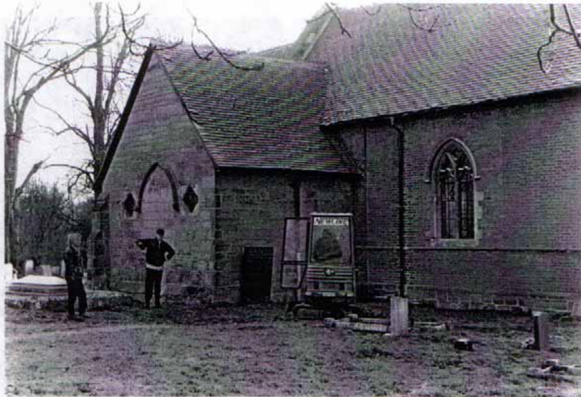
Fig. 5: Evaluation Area before Excavation
